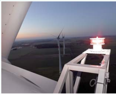
W-Red light on an E-82 at Schweringhausen, Lower Saxony.
