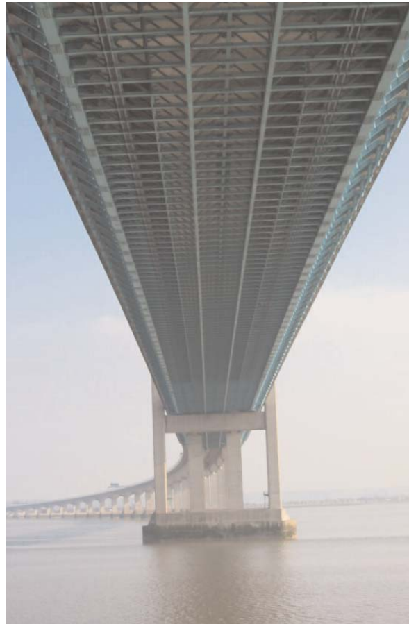
A view from beneath the new Severn Bridge where one of the Biral HSS VF-500 fog detectors is positioned.
